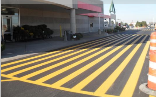
FDR with Cement Slurry & New Pavement
